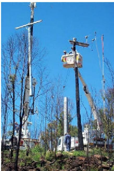
Installing the new steel poles, adjacent to a burnt out wooden pole
