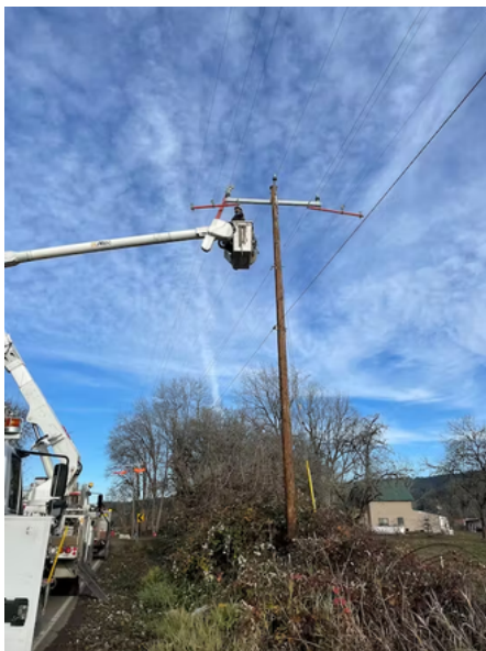
A utility worker clips in a new conductor to a distribution crossarm. Long-term system hardening projects — including overhead-to-underground conversion, covered wire and intelligent reclosers — are critical to the reduction of wildfire risk.
