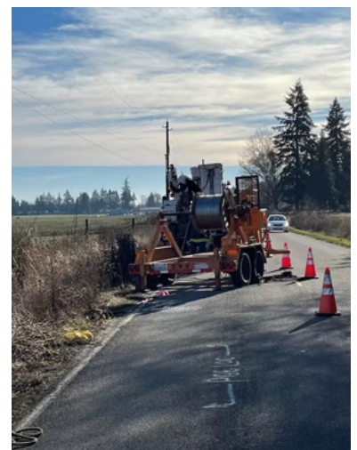
New conductor ready to install in the Willamette Valley.
