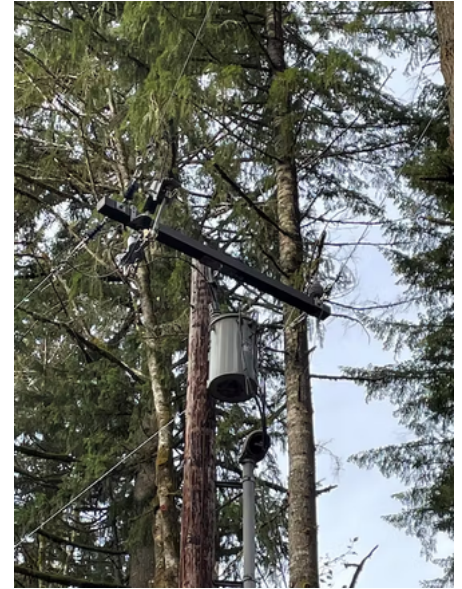
A power pole equipped with a new conductor, X-arm and cutouts.
