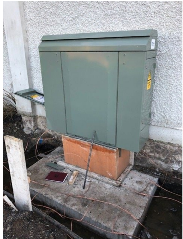
Fig. 5 Prototype Sidewalk Transformer 200kVA
