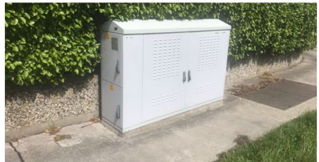
Fig. 5 Prototype Sidewalk Transformer 200kVA
