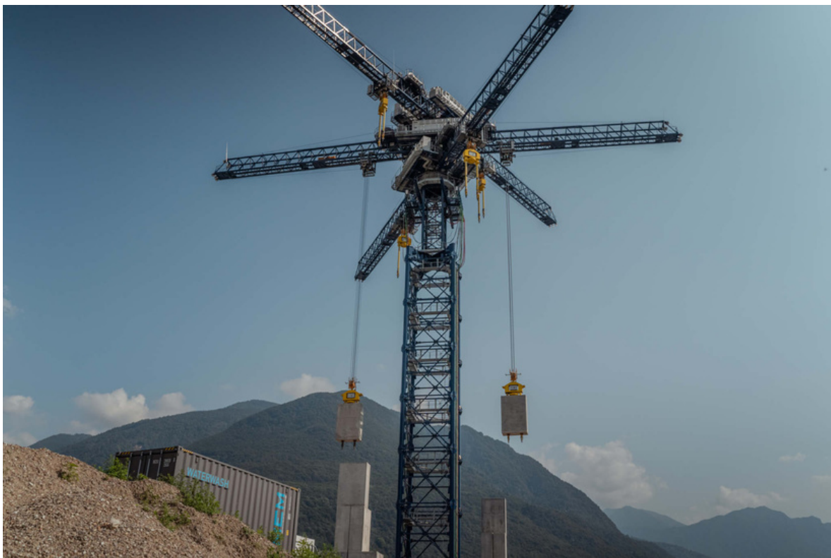
Energy Vault's working model of its technology in Switzerland generates electricity when the blocks fall to the ground. CREDIT:ENERGY VAULT
