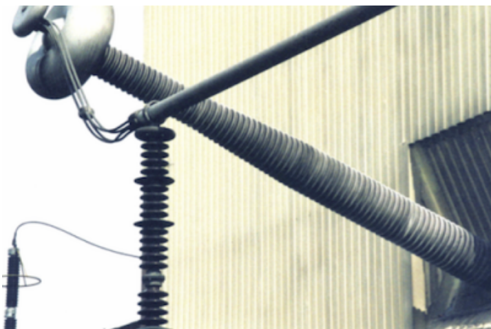
Uneven pollution distribution on porcelain-housed wall bushing makes it more vulnerable to flashover under wetting.
