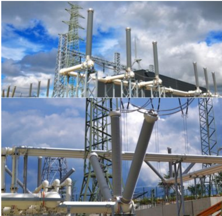
Gas-insulated bushings with composite housings in Belgium, Czech Republic and Korea.
