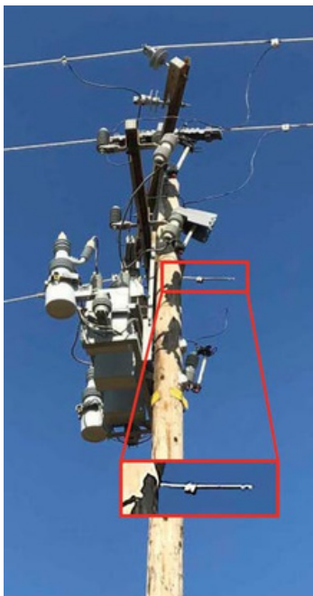
Broken conductor at capacitor bank.
