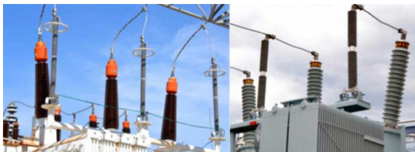
Optimizing OIP design has allowed reduced diameters of external porcelain housings.
