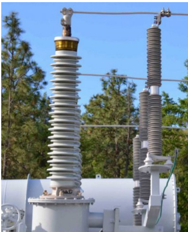
Among subtle improvements in OIP bushings has been improved sight glass design for visual monitoring oil level.
