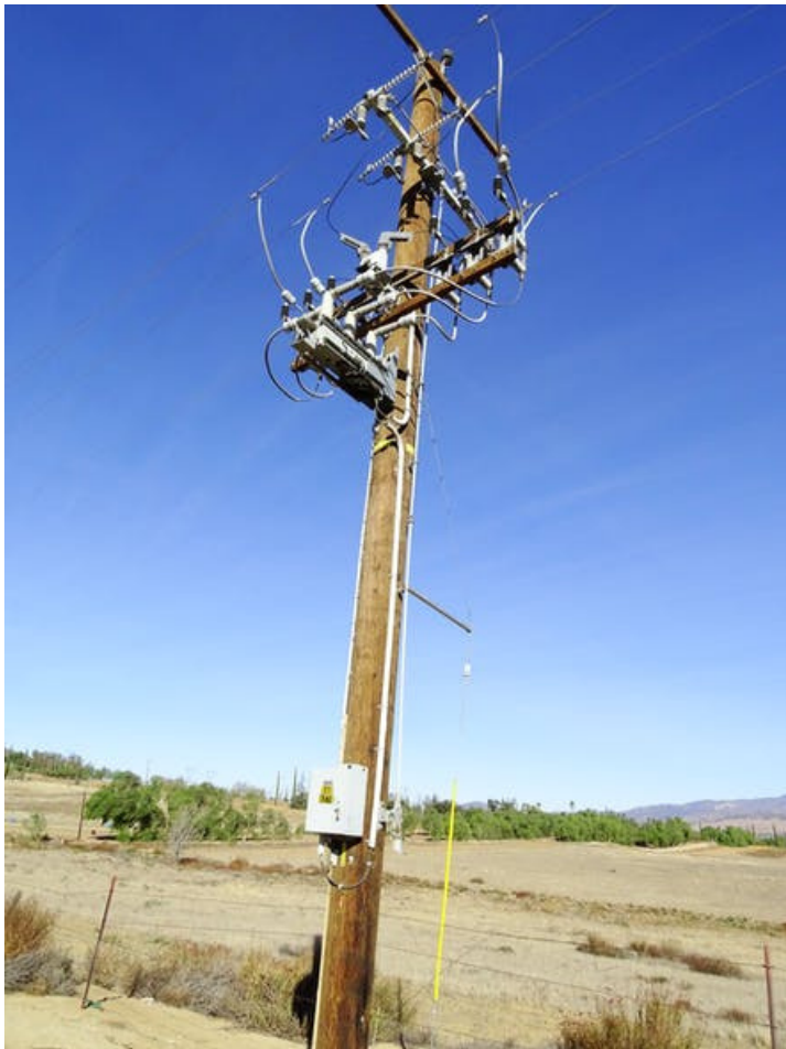
Distribution overhead pole with automatic recloser and control device.
