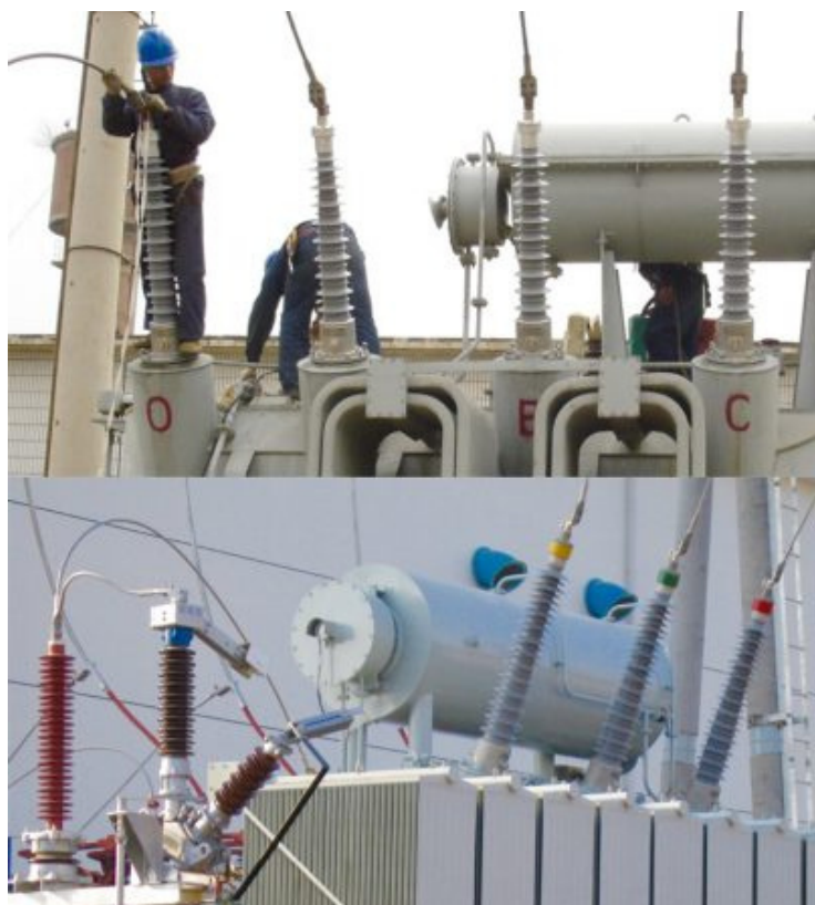
Dry RIS type bushings installed in China at 66 kV and 110 kV.
