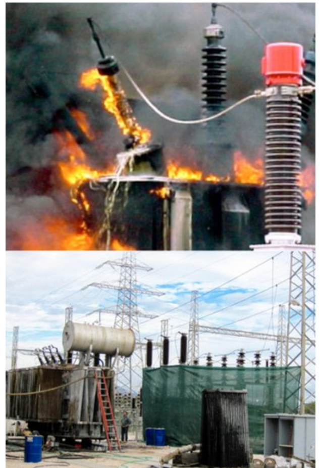
Catastrophic bushing failure means expensive repairs or even total loss of transformer.
