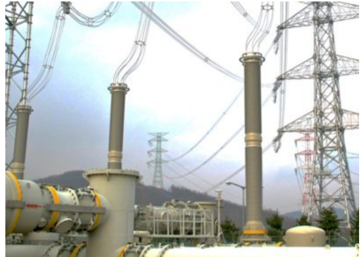
Gas-insulated bushings with composite housings in Belgium, Czech Republic and Korea.
