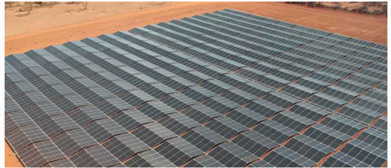
ARENA's Solar 30 30 30 goal is to realise solar module efficiency of 30 per cent and an installed cost for solar farms of 30 cents per watt by 2030 (Image: Supplied)
